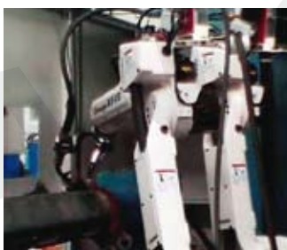
Girder robot welding
